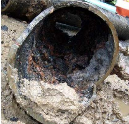
***Existing unlined cast iron water main with significant scale buildup.***
