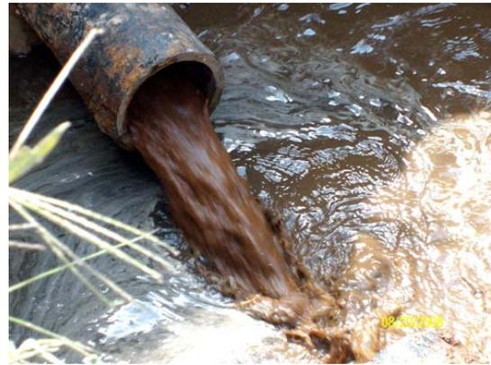
***Water Flowing from Water Main During the Cleaning Process.***
