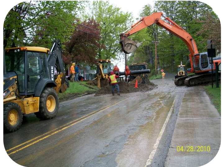
Route 5 Water Main Construction
