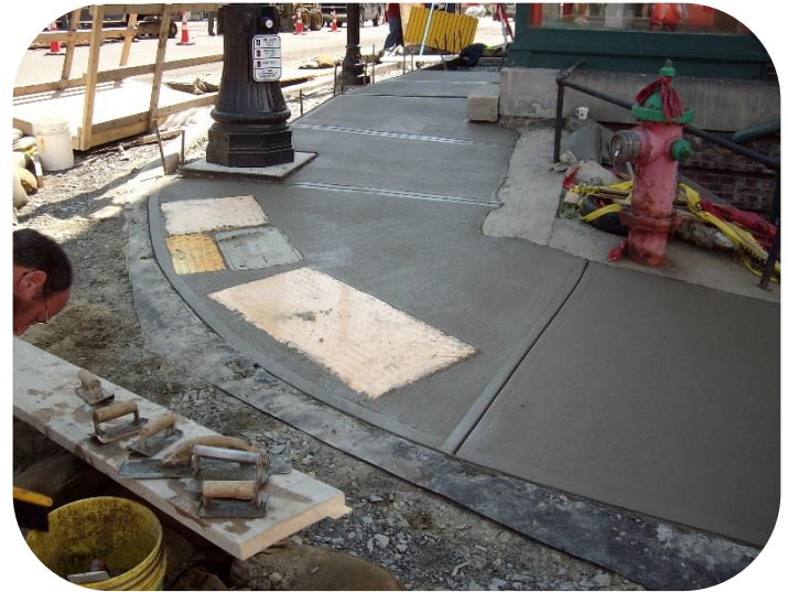
Sidewalk In Progress
