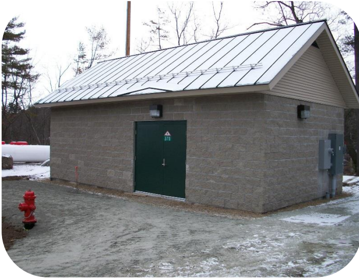
Exterior View of the Commonwealth Pump Station
