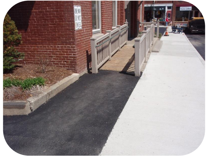
Sidewalk Along West Side of Depot Square at the Merchants Bank
