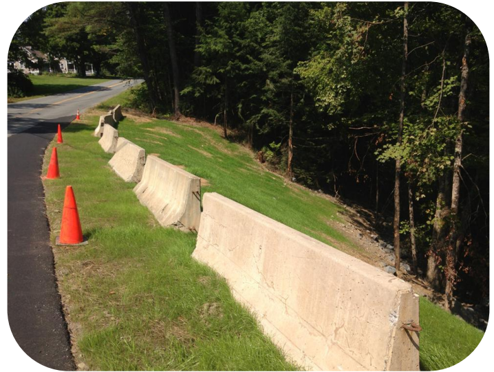
Stabilized bank pending permanent repairs
