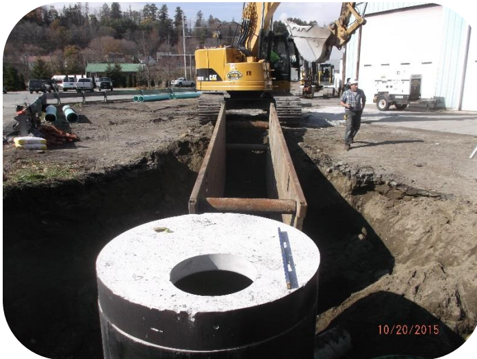
New Sewer Main Installation, Eliminating a CSO Connection
