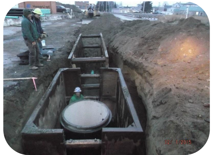
Installation of new 8" SDR-35 PVC sewer main
