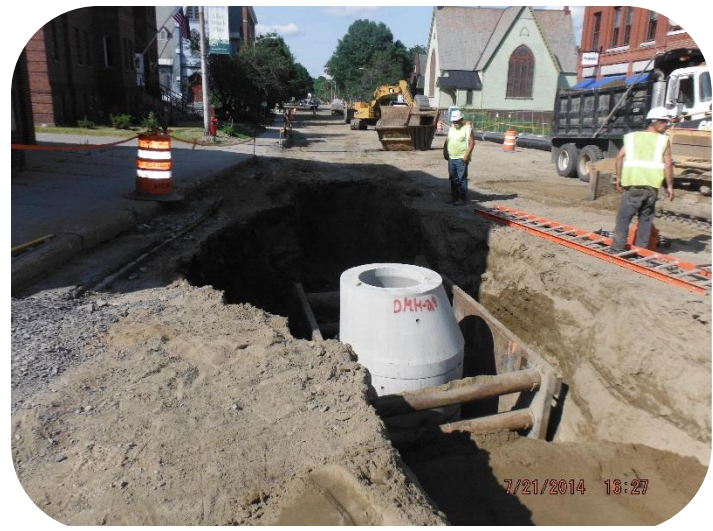
New Storm Drain Installed as Part of the Project
