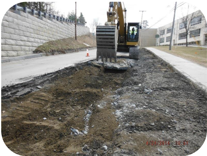
Removal of Existing Concrete Roadway and a Full-Width Road Reconstruction
