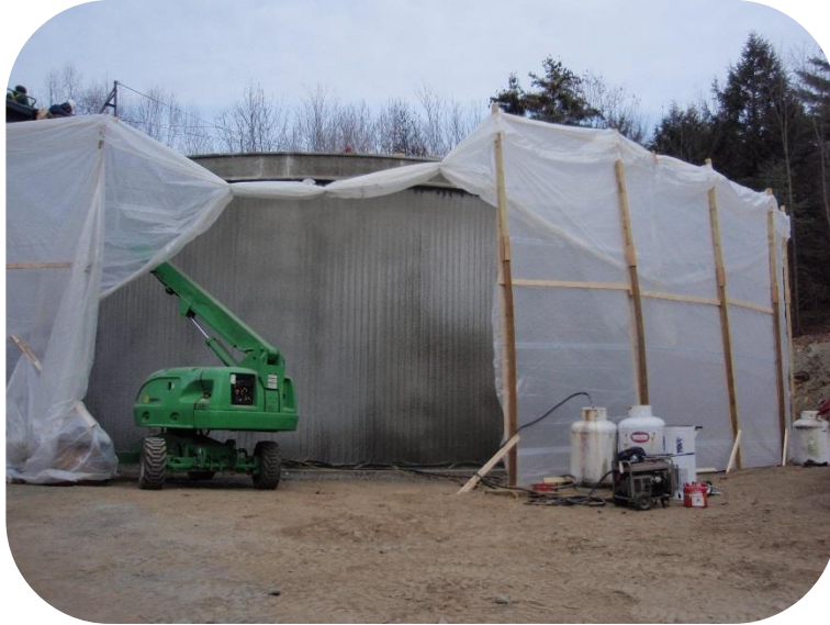
Precast-Prestressed Tank Prepared for Wire Winding During Winter Conditions.
