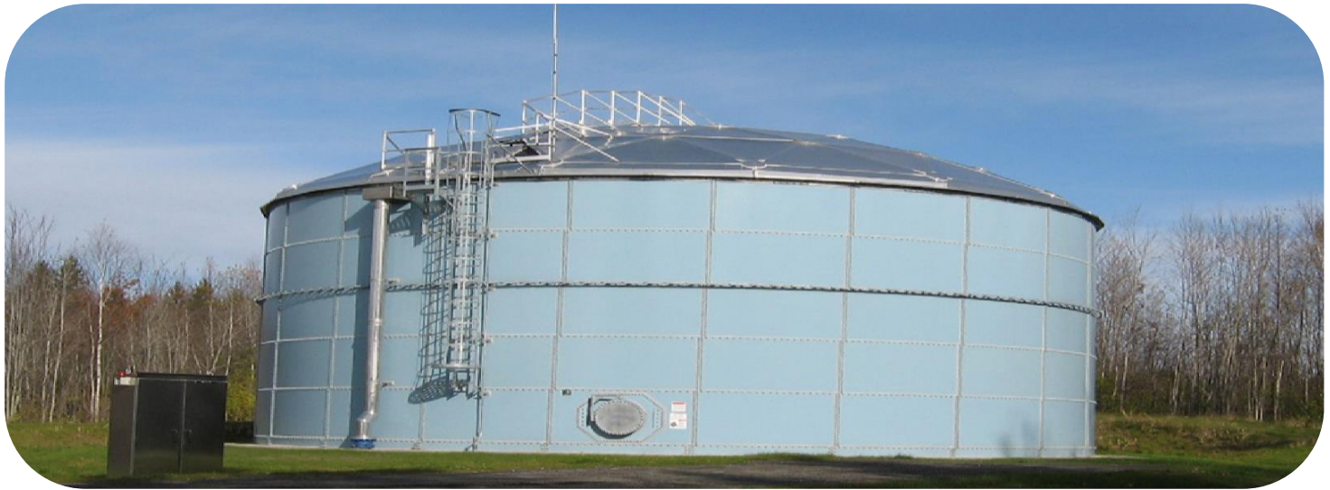
Airport Road Water Storage Tank
